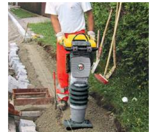
Exact unit guiding – important during compaction in border areas.
