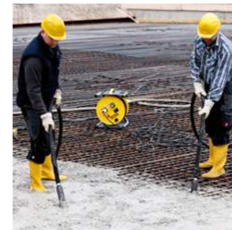
Dependable and sturdy: internal vibrators by Wacker Neuson are indispensable on many construction sites.
