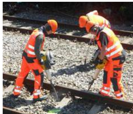
Gasoline breakers BH40 and BH55rw are specially optimized for maintenance work in railway construction.
